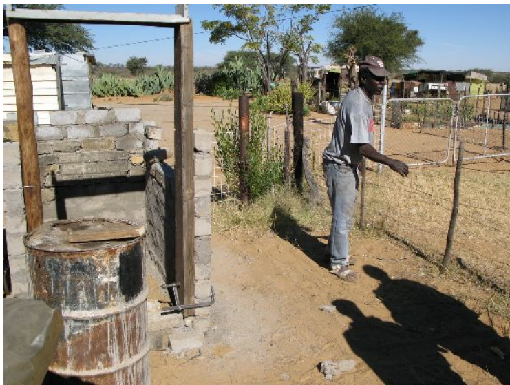
Photo 14: Joseph Ganeb building a latrine
